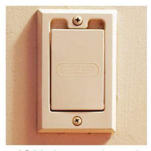
Located on apartment wall. Pull the door open, push vacuum hose into port and system starts automatically. When completed vacuuming, carefully pull hose out of port.
