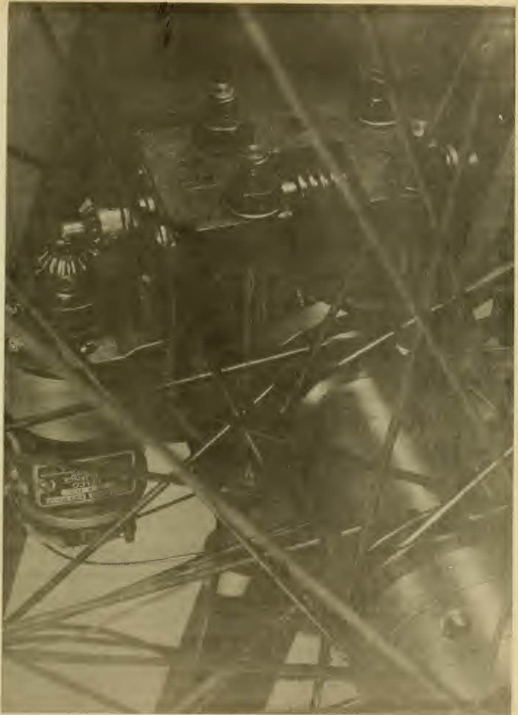
Figure 7 Close Up View, Differential System
