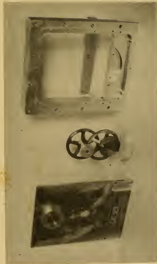
Photograph 6-A Component Parts of Gear Box, Rear View
