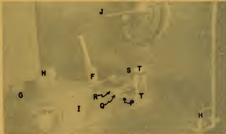
Photograph 4-b Detailing Point of Main Motor Drive Shaft and Shell Crank Assembly
