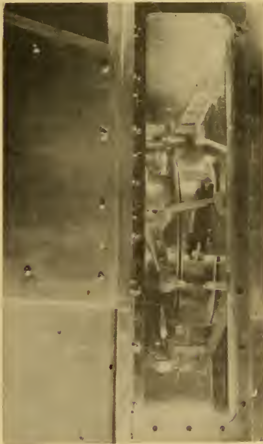
Photograph 6-C Interior of Reel Chamber seen via Inspection Mirror
